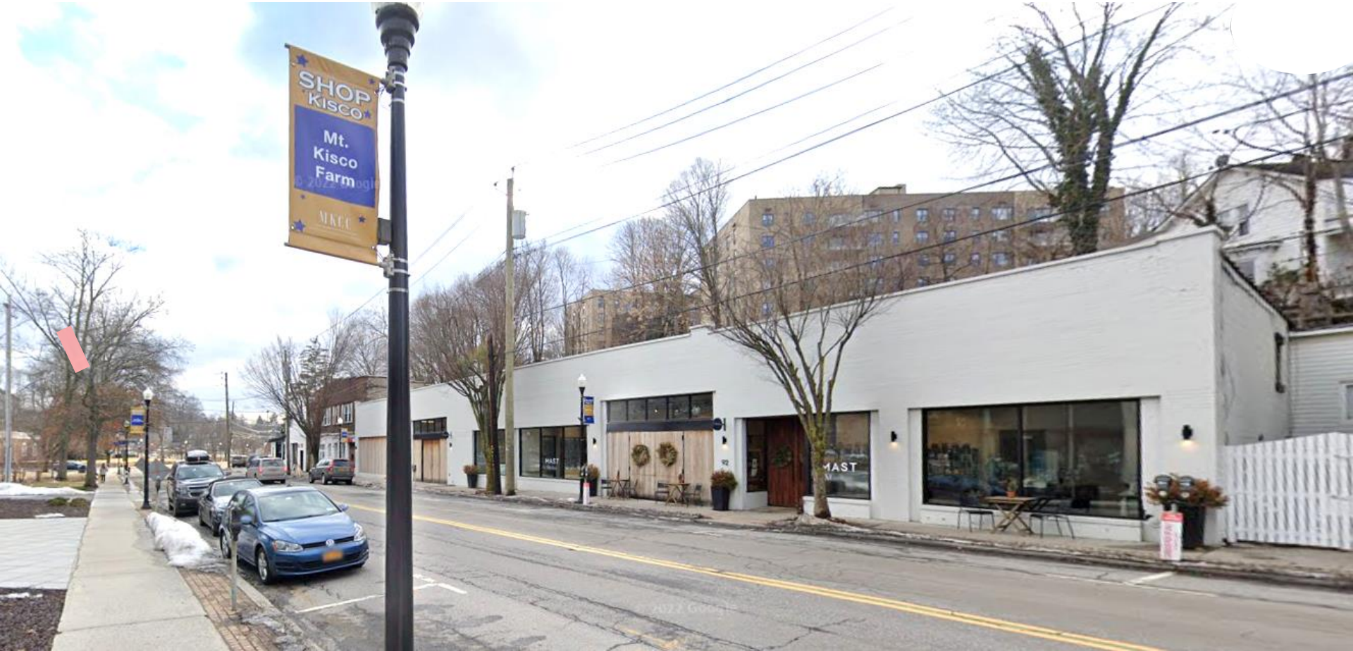
Facing South on South Moger Avenue
