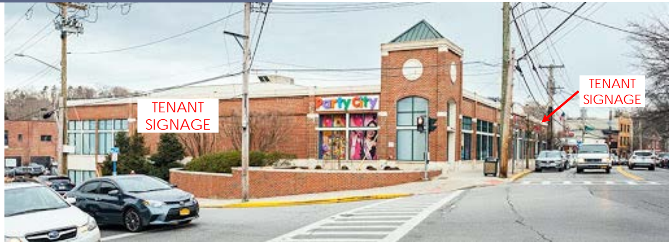
At signalized intersection of East Main and Green Streets facing northwest toward Metro-North
