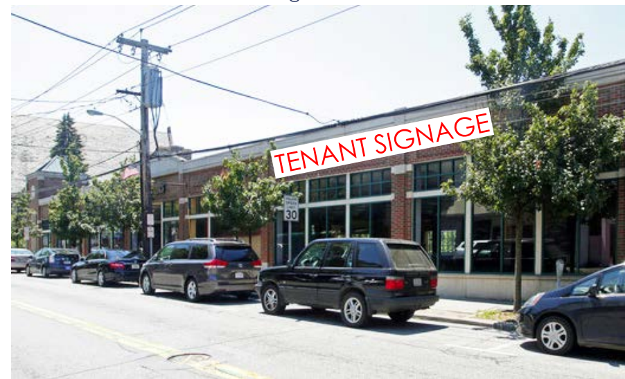
Front entrance facing southwest toward Green Street
