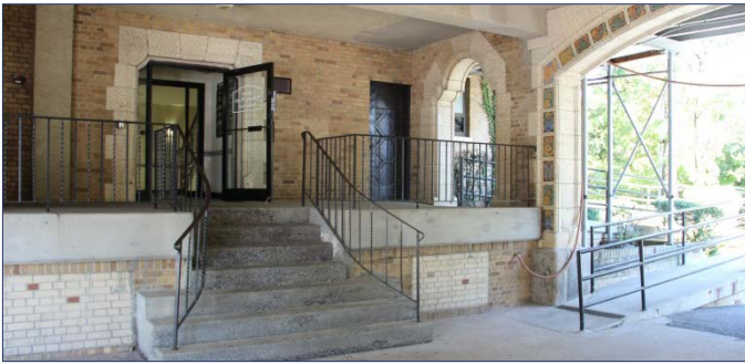
Drop Off Right in Front of Entrance
